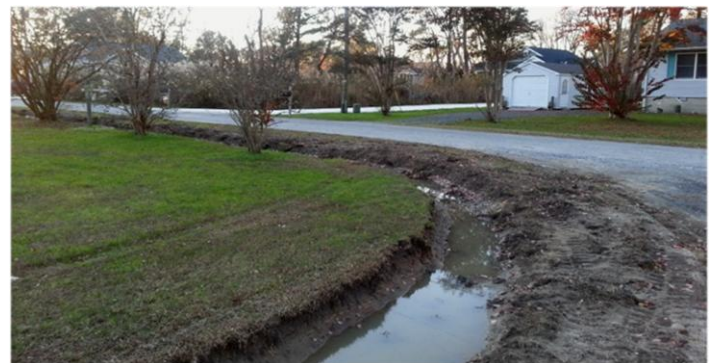
Trenching in Progress
