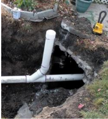
Typical clean-out pipe with cap
